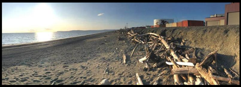
Erosion of berm fronting Shaktoolik (red) Area of erosion: 110,000 sq. ft Amount of erosion: 350,000 cubic ft
